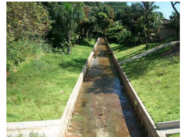
Canal Mirandinha – Boa Vista – RR Drainage canal
